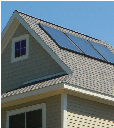
Solar panels capture the sun's energy, which is then used to heat your water.
