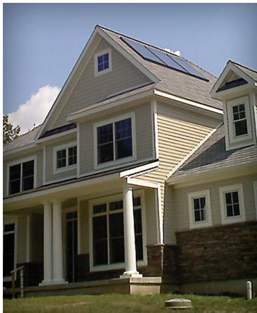
The Radiant Store performs more residential installations than any other NYSERDA-eligible installer.
